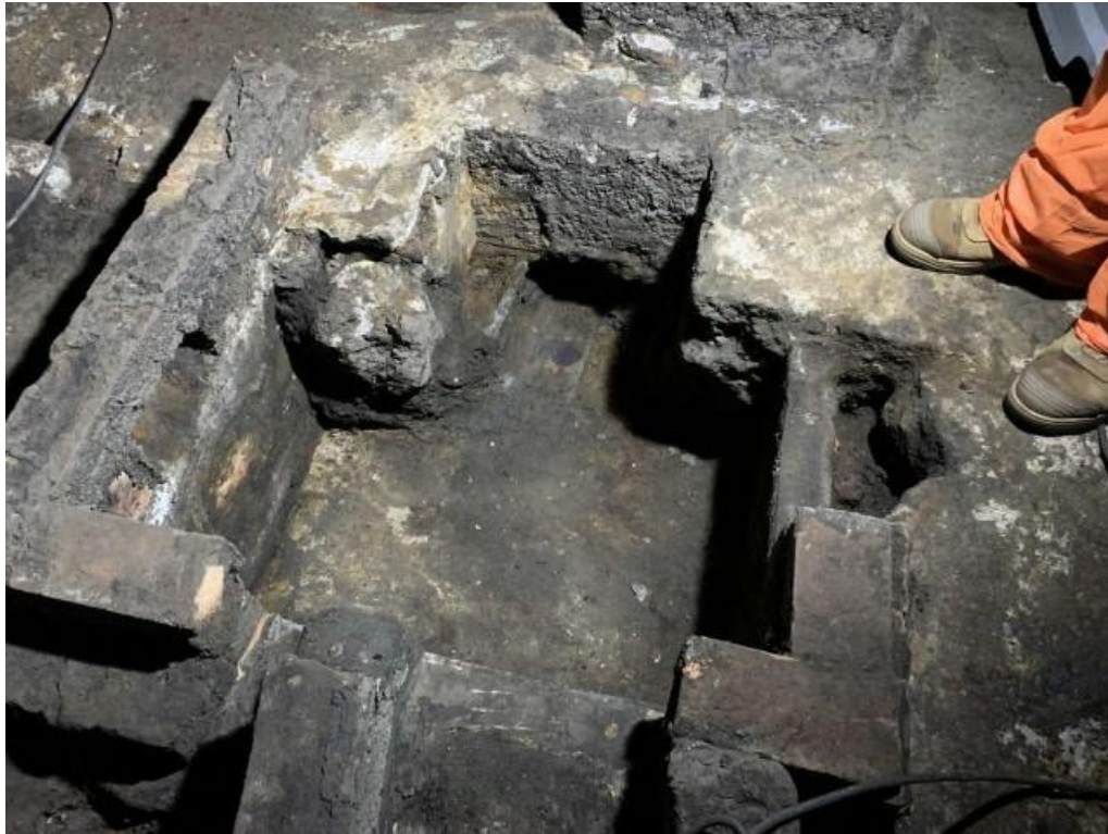
Figure 53. Engine Room sub-floor cavity 2020. Central sump pit with drains to exterior.
