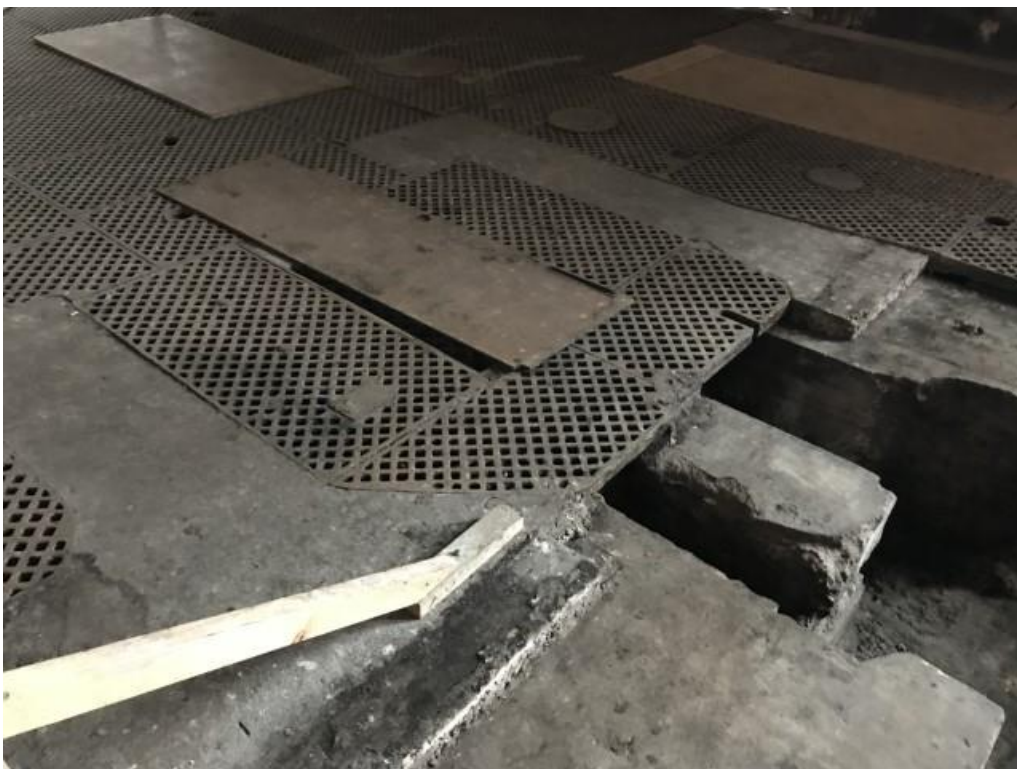
Figure 36. Engine Room – Detail, Cast Iron Floor grates.
