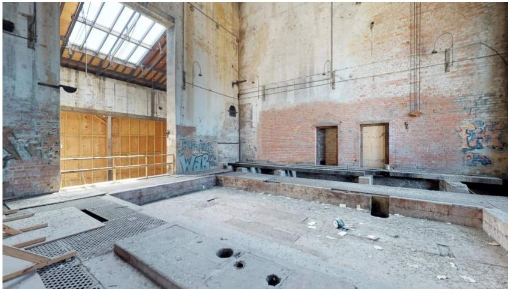
Figure 31. Engine Room, looking north east, large opening through to generator room (currently sealed temporarily to encapsulate asbestos hazard).
