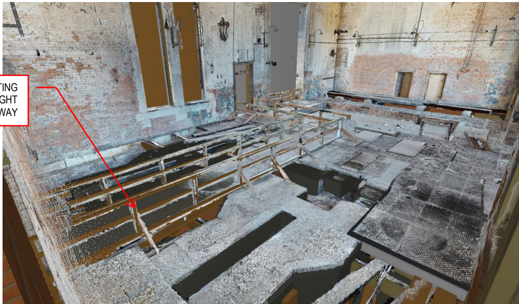
Figure 65. Existing CHEH Engine Room, perspective view looking east, 3D Architectural Model /Point-Cloud scan. Many large openings are present across the floor plate, loose timber beams and panels scatter the floor, and a lightweight contemporary timber walkway spans across the non-trafficable floor structure.
