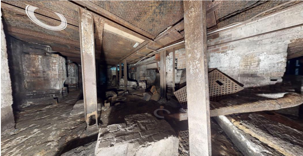
Figure 58. A very deep sub-floor cavity is present below the grates, which has been cleaned of asbestos as best as possible.
