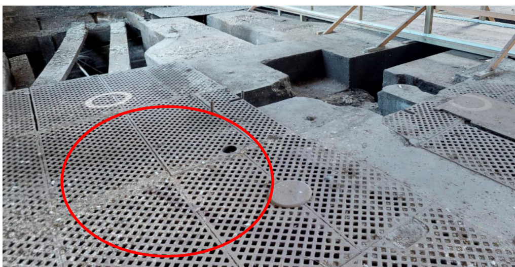
Figure 57. The cast iron floor grates present an asbestos hazard, with their porous surface containing remnant fibres despite previous cleaning in the room. Note also the large cavities present across parts of the floor. The project hygienist has described that it would be implausible to fully clean the grates of asbestos in-situ, given the myriad openings and porous surface.
