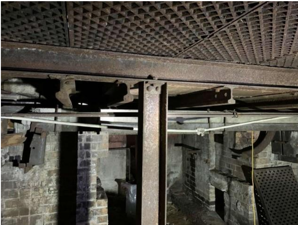
Figure 52. Engine Room sub-floor cavity 2020. Column and framing to cast iron floor grates.
