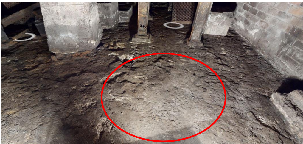
Figure 59. The solidified base surface however presents an asbestos hazard, with detectable asbestos physically embedded within the surface material.
