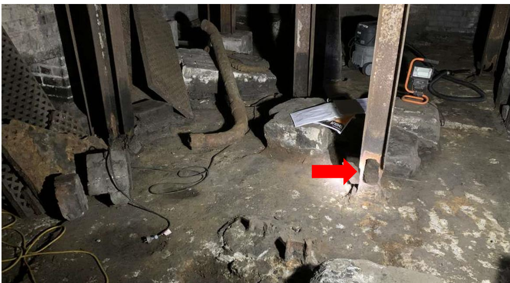
Figure 60. Typical photo of steel columns supporting the cast iron grates. All are suffering extreme corrosion at their base with over 90% section loss, meaning that the grates above are non-trafficable and at significant risk of collapse.
