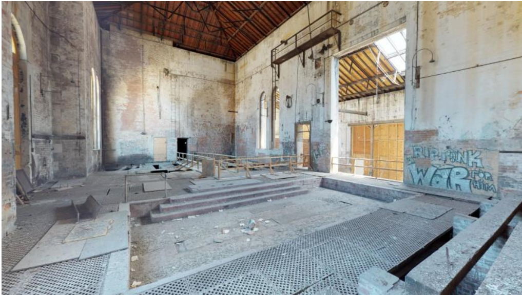
Figure 29. Engine Room 2018, prior to first stages of asbestos removal works, looking west. All openings through to generator room and other rooms are currently sealed temporarily to encapsulate asbestos hazard within the Engine Room.
